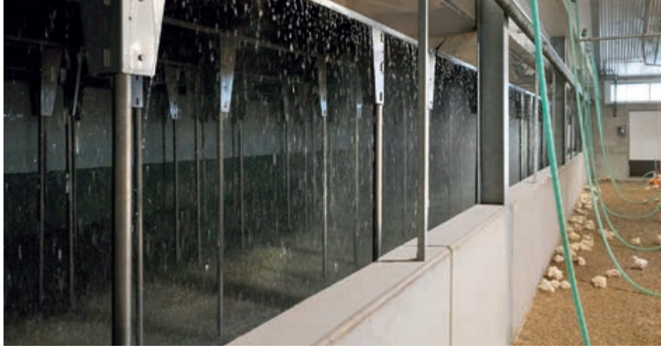
Pollo-M is easily accessible; constant humidification keeps the filter element clean
