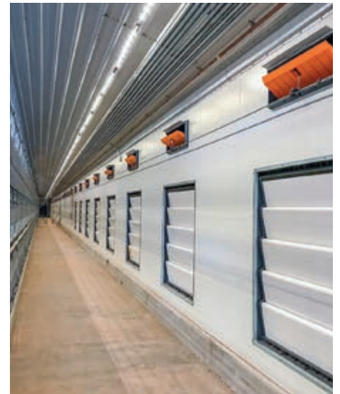
Aviary house with CombiTunnel ventilation, using CL 1911 F wall inlets and MVT shutters
