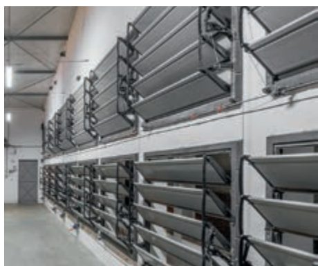
MultiVent 17 M in the gable wall for tunnel ventilation
