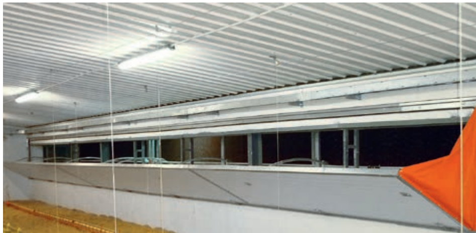
Broiler house with tunnel door, opening into the barn
