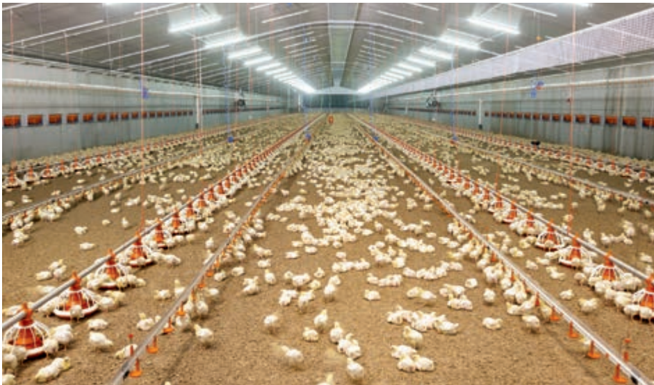
Typical broiler house in Northern Europe with fresh air supply through CL 1911 F wall inlets
